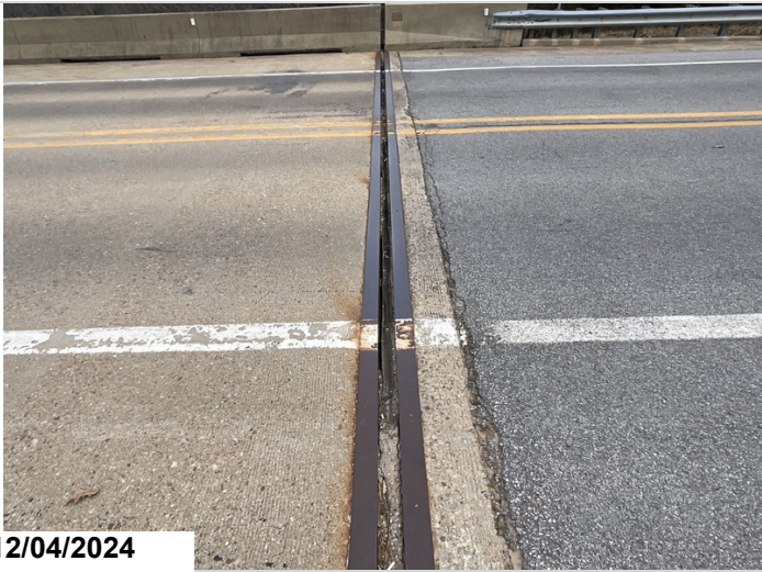
Abutment 1: Adhesion failure/leakage: 43LF CS3
