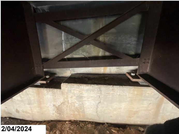
Abutment 1: has vertical cracks and efflorescence.
