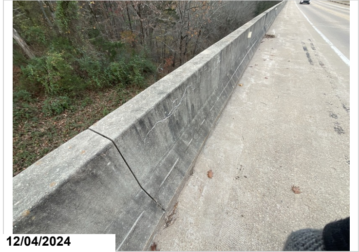
Areas of heavy efflorescent map cracking to Parapet walls on Left and Right sides.152LF CS3
