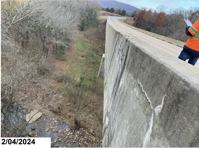
Areas of heavy efflorescent map cracking to Parapet walls on Left and Right sides.152LF CS3
