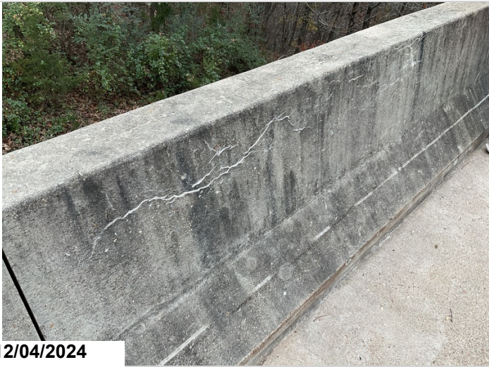
Typical efflorescence
