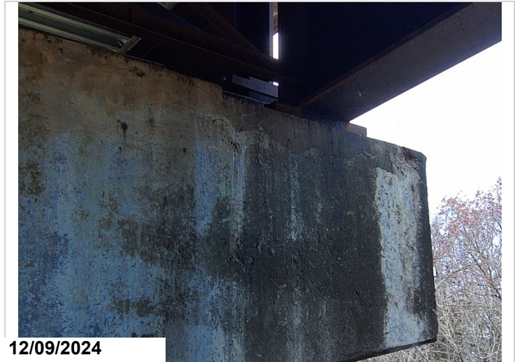
Bent 2: Backside Right: Spall. 1LF CS3
