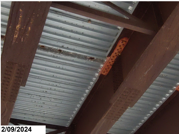
Areas of rust to stay in place forms above field splices at all spans.
