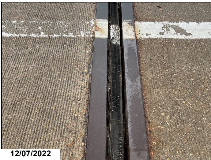
Pourable joint seals are deteriorated and leak.
