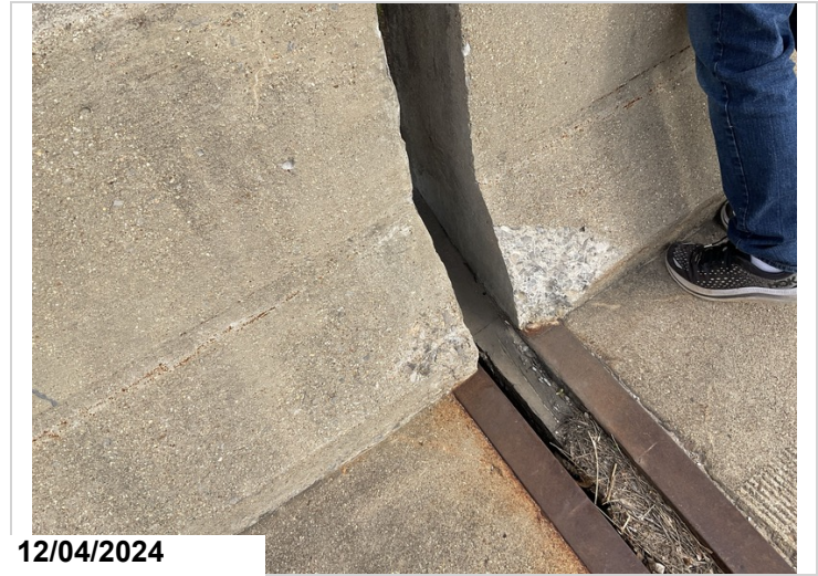
Bent 2, right: has a spall at the joint. 1LF CS3
