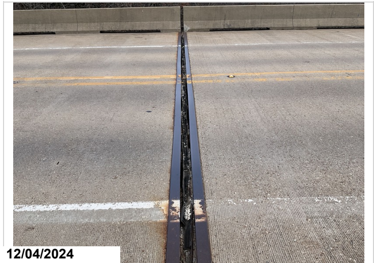
Bent 1: Adhesion failure/leakage. 43LF CS4
