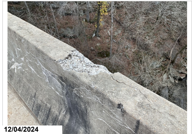
Span 2: Left rail: Spall. 1LF CS3
