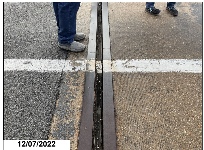
Pourable joint seals are deteriorated and leak.
