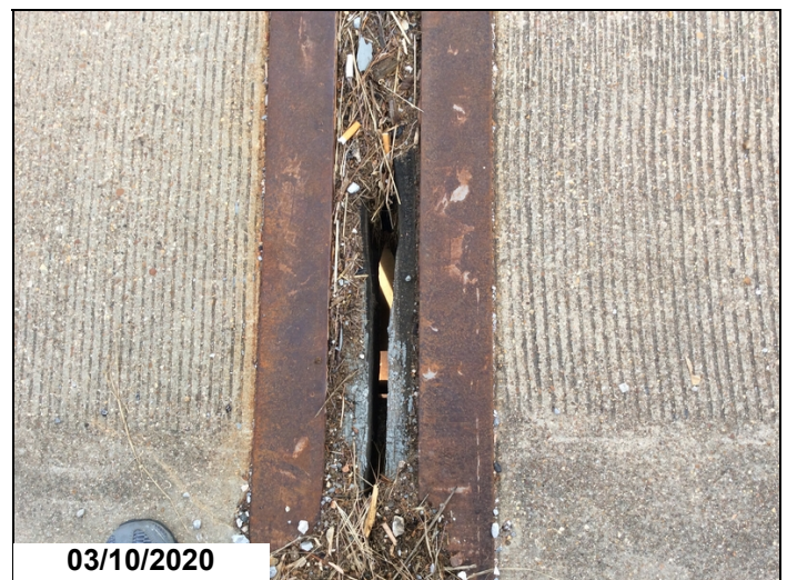
Pourable joint seal is losing adhesion @ Bent 2.
