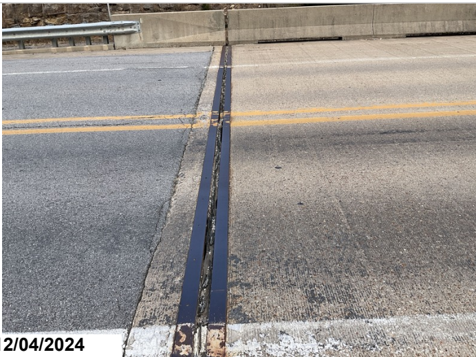
Abutment 2: Adhesion failure/leakage: 43LF CS3
