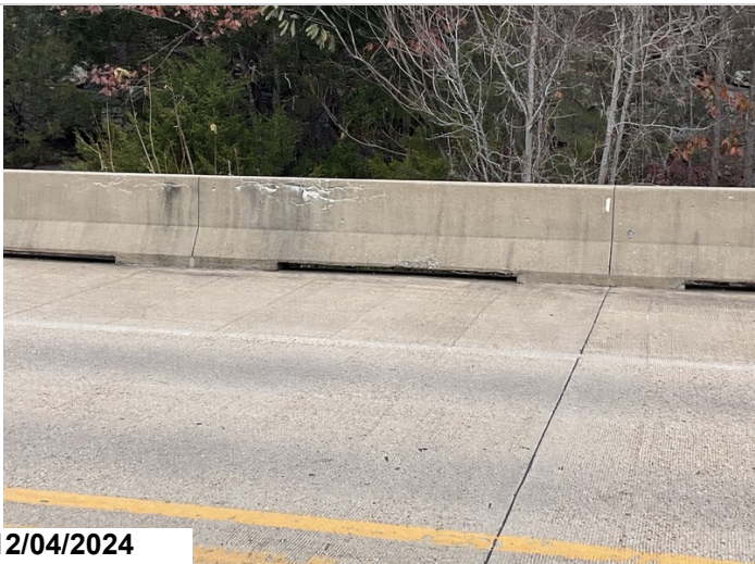
Span 4: Right: Spall. 2LF CS3
