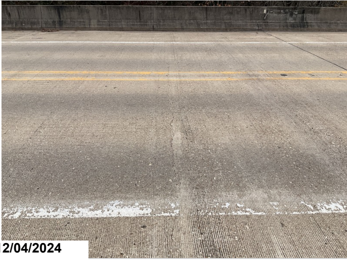
Span 1: transverse cracking. 80LF CS3
